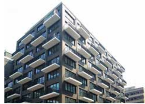
Residential Quarter at Alexanderplatz, Berlin 2012-2015, completed Client SONUS City GmbH & Co. KG GFA 40.700 m 2 DGNB Gold certificate
