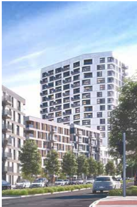
Grand Central, Düsseldorf/Germany 2015-2021 Client Catella Property GmbH, Düsseldorf GFA 100.000 m 2 Use 665 flats, 2 kindergartens, retail
