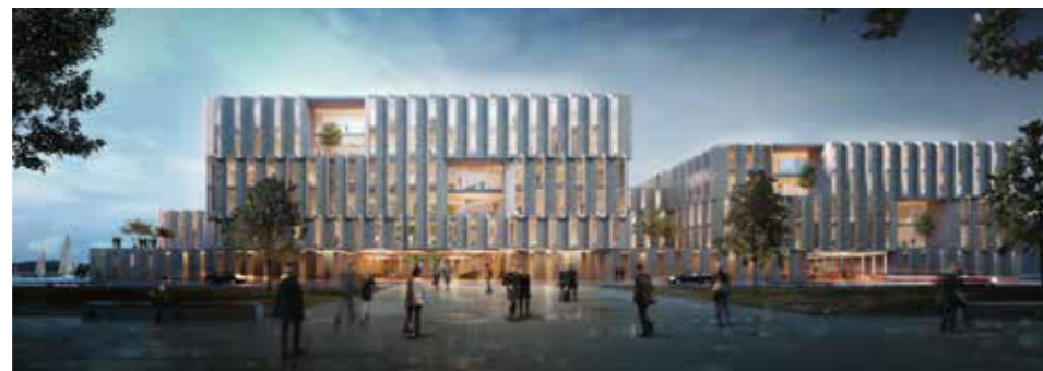
ATS Headquarters, Yekaterinburg/Russia 2015-2020 Client ATS, Yekaterinburg GFA 30.000 m 2
