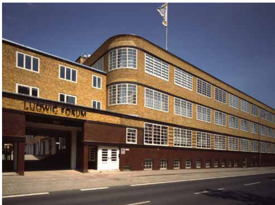
Museum Ludwig Forum, Aachen/Germany 1988-1991, completed Client City of Aachen GFA 7.000 m 2
