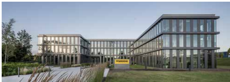
Headquarters Turck, Mülheim Ruhr/Germany 2013-2016, completed general planner Client Turck GmbH und Co. KG, Mülheim/Ruhr GFA 4.200 m 2
