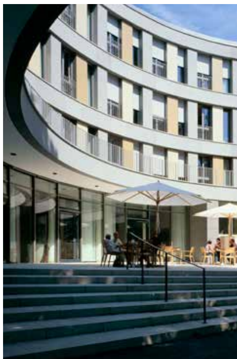
Nursing Home & Kindergarten, Duisburg/Germany 2004-2006, completed Client Franz Haniel & Cie. GmbH, Duisburg GFA 5.200 m 2 nursing home, 600 m 2 kindergarten
